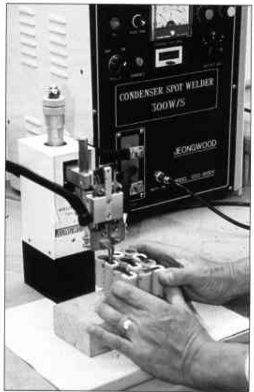
Photo.3: NiCad Batteries being assembled on the Akkupak assembly line using an electronically controlled spot welder
